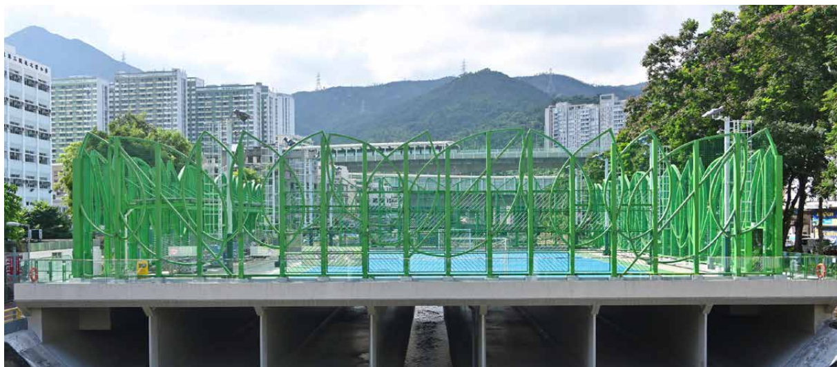
In an innovative move, the five-a-side Tai Wai Soccer Pitch was built over an existing nullah.
