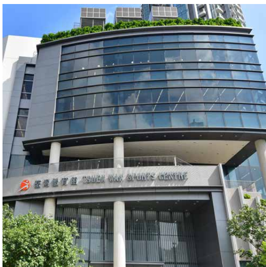
The new Tsuen Wan Sports Centre opened for public use in October 2018.
